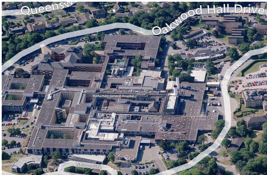
Fig. 3.2 Rotherham Hospital, Rotherham, UK - English Streamer demonstration project
