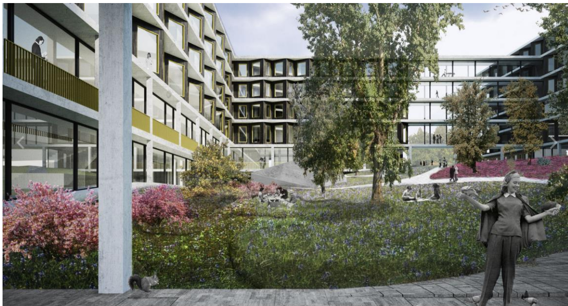
Fig 3.8 Jan Portaels hospital, Vilvoorde, Belgium (image by NU architectuurstudio)
