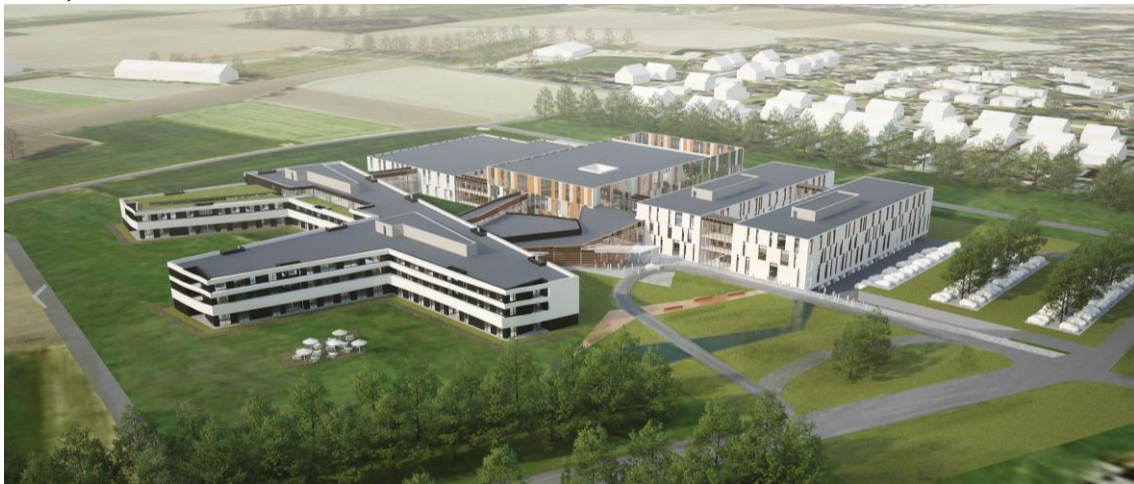
Fig 3.12 Maas en Kempen Hospital, Maaseik, Belgium (image by DjGA)
