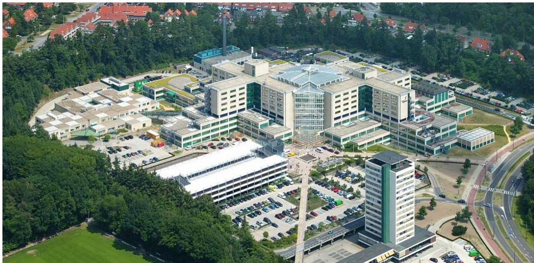
Fig. 3.6 Rijnstate hospital, Arnhem, The Netherlands - Dutch Streamer demonstration project (image by Rijnstate)
