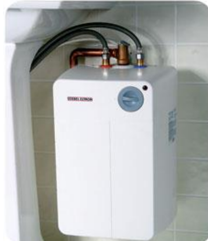
Figure 18 Electrical boiler
