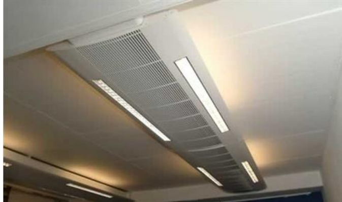
Figure 76 Chilled beam
