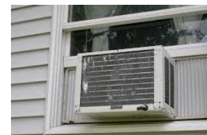
Figure 67 Outside unit/condenser
