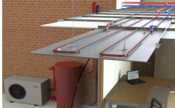
Figure 73 Radiant ceiling panel s installation
