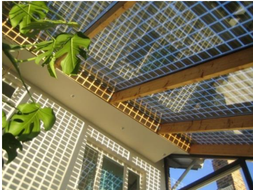
Example of overhang glass with integrated PV panels.
