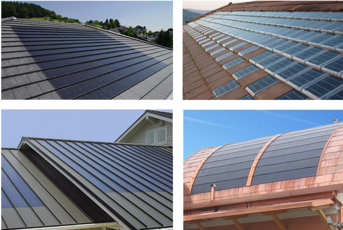
PV panels integrated in a pinched roof
