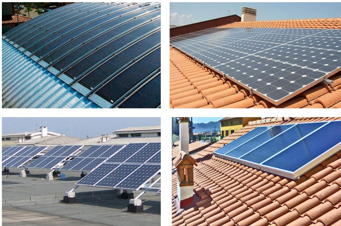
Figure 2 PV panels can be installed on different type of roof.
