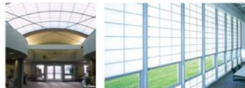
Encapsulated granular aerogel: (Available from companies such as Kahwall + Xtralite)
