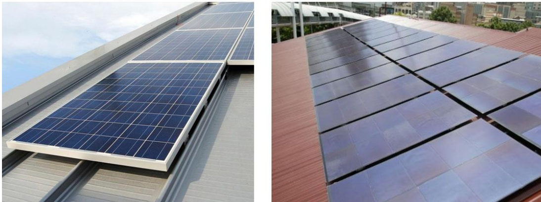
Figure 1 Example of PV panels.
