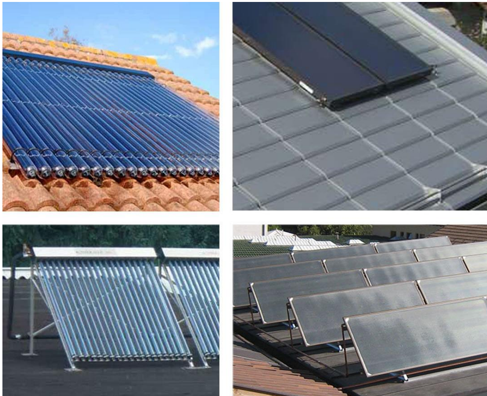
Figure 2 - Application on roofs
