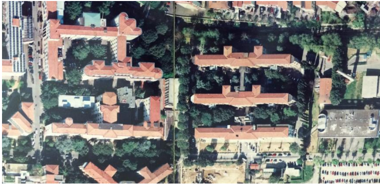
Figure 6: San Luca complex aerial view before the demolition of two buildings
