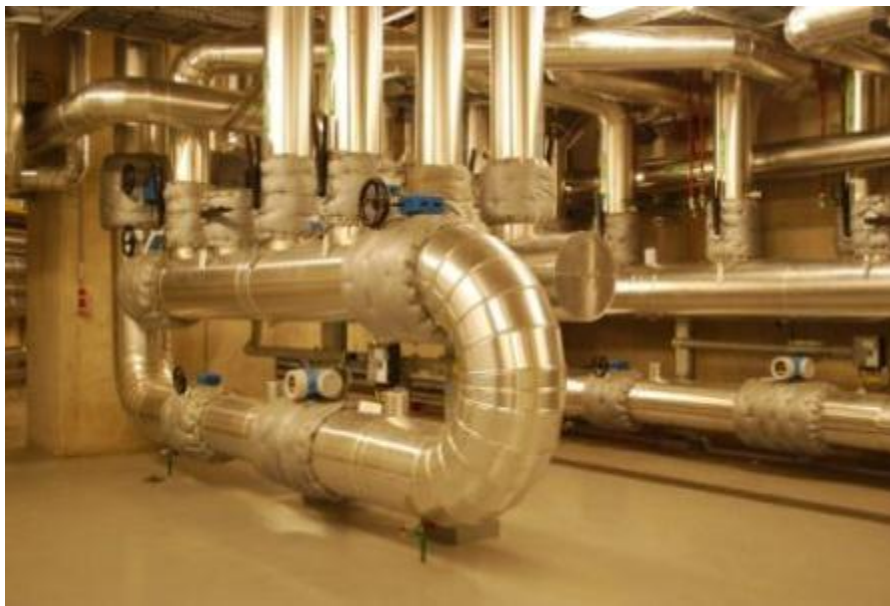
Figure 17 Hot water distribution
