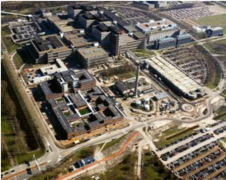
Figure 19 Overview AMC area (power station in the middle – below)
