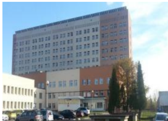
After thermal modernization
