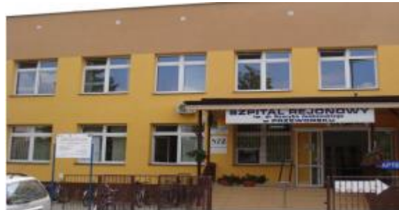
After thermo modernization
