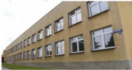
Before thermo modernization
